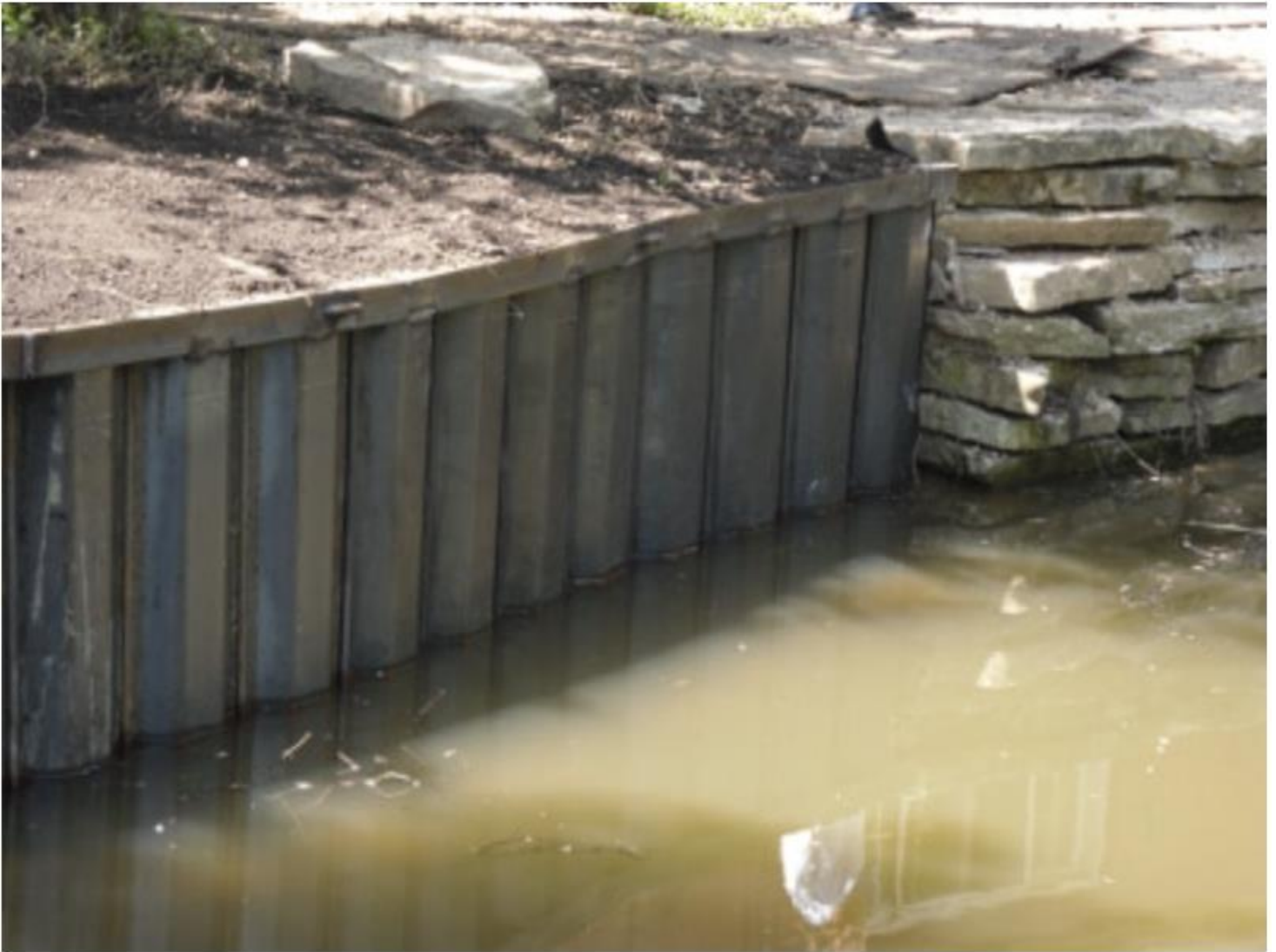
Example of an intact retaining wall
